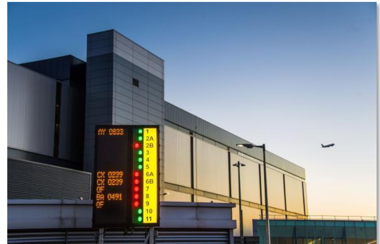
Terminal 3 Integrated Baggage facility
