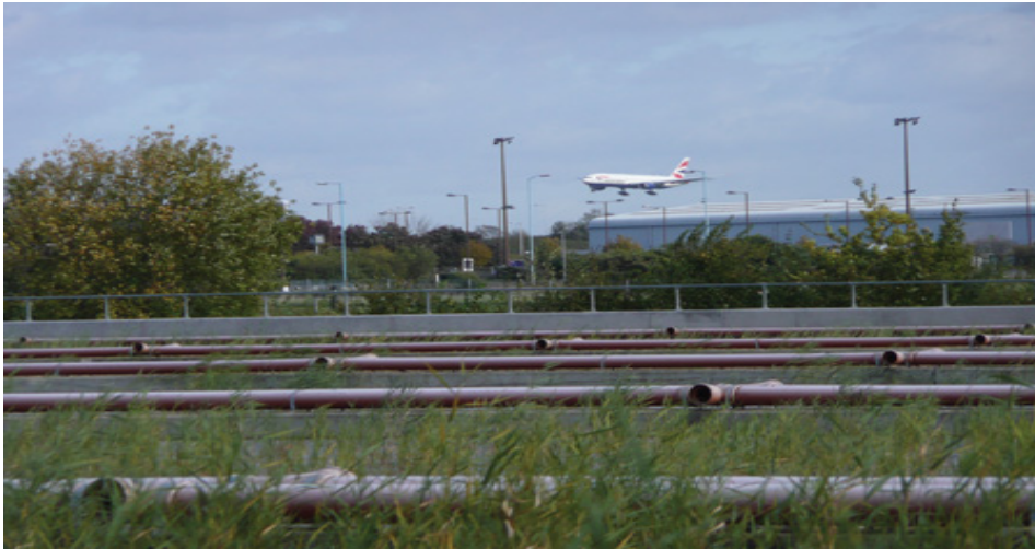
Figure 5.46: Existing reed bed at Heathrow's Mayfield Farm Treatment Facility
