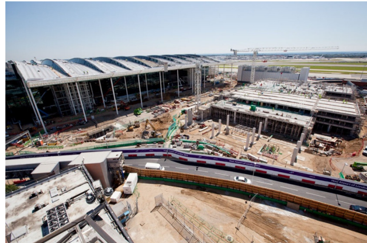
Terminal 2 site – July 2012
