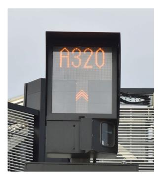
4.2.5 If an aircraft is present on stand, or partially on stand, prior to the activation of the SEGS the aircraft may be recognised/identified by the system as an obstruction and guidance will not start. In these circumstances the aircraft will need to be marshalled onto its stopping point.
