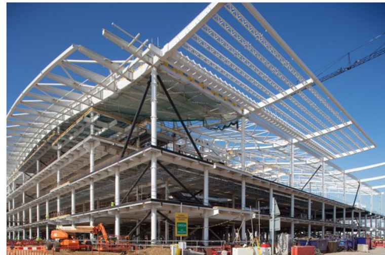
Terminal 2 site – March 2011
