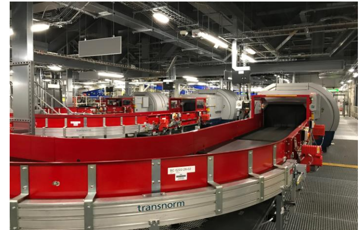
T5 Hold Baggage Screening replacement
