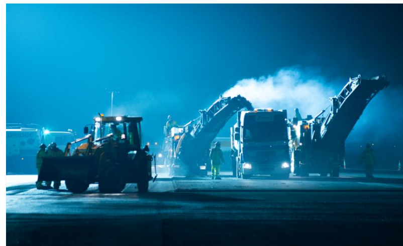
Night time resurfacing of the northern runway
